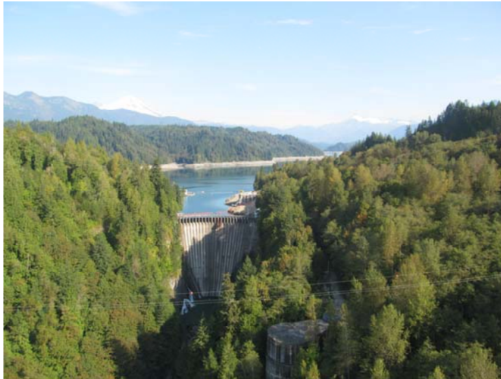
Lake Shannon and Lower Baker Dam (constructed 1925) Photo by John Chandler, Puget Sound Energy
