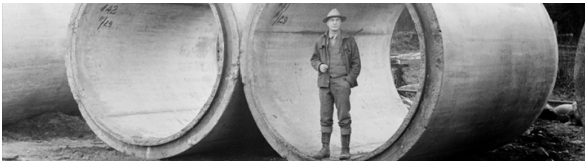
Cedar River Pipeline at Landsburg, man posing in pipe, 1929
