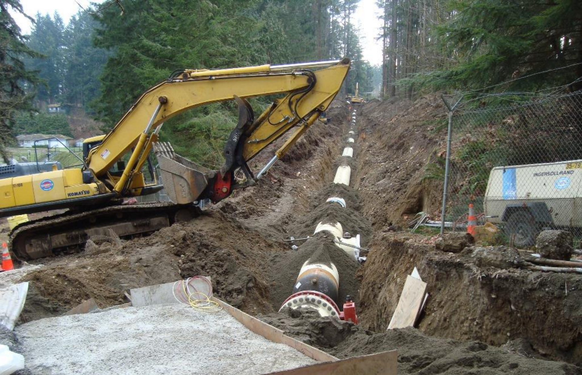
McAllister Wellfield Pipeline - Connecting at Springs
