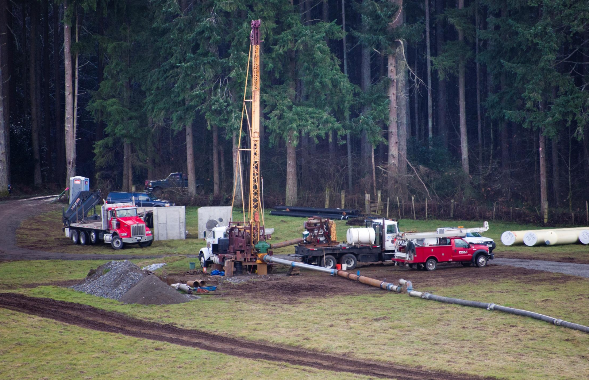
Drilling new 24-inch well at McAllister Wellfield
